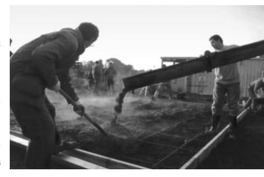
The use of WRDA 64 produces a plastic concrete that is more workable, easier to place and more finishable than plain or other admixtured concrete. In the hardened state, WRDA 64 concrete has higher compressive and flexural strengths at all ages than untreated or conventional admixtured concrete.
